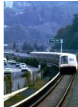
Cover Photo: San Francisco's Bay Area Rapid Transit (BART) system. Harmon received a contract, including all options, valued at $45 million in February 1998, to design and install a revolutionary communications-based automatic train control system on BART's highest density lines. The new system will employ an innovative radio technology that was developed by Hughes Aircraft Company (now Raytheon Company) for the U.S. military forces to track vehicles and personnel on the battlefield.
