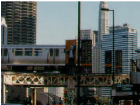
Harmon is supplying a new, electronic signal and control system for Chicago's "Green Line," one of four rail transit routes operated by The Chicago Transit Authority.
